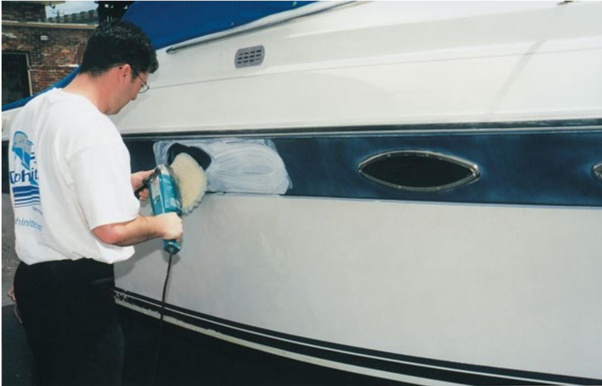
The outer surface of a fiberglass boat is normally a special resin called gelcoat. Gelcoat has little structural value — the underlying laminates of resin-saturated glass fabric provide that — but gelcoat protects the hull and gives it its color and shine.
